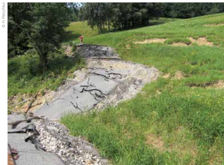
Rotational landslide with deformed agricultural road in Stössing, Lower Austria in June 2009
